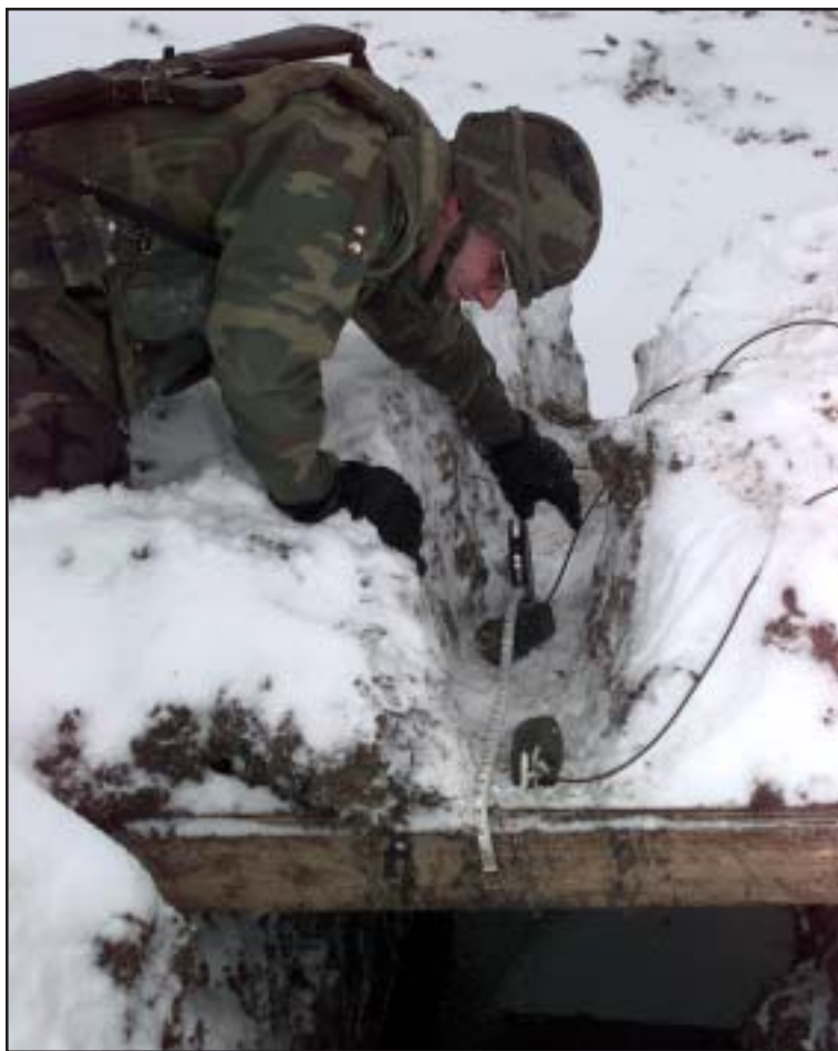
Specialist Mark Costa, 2nd Platoon, Company C, 20th Engineers, measures spacing for charges for detonation of a two-man fighting position with overhead cover.
