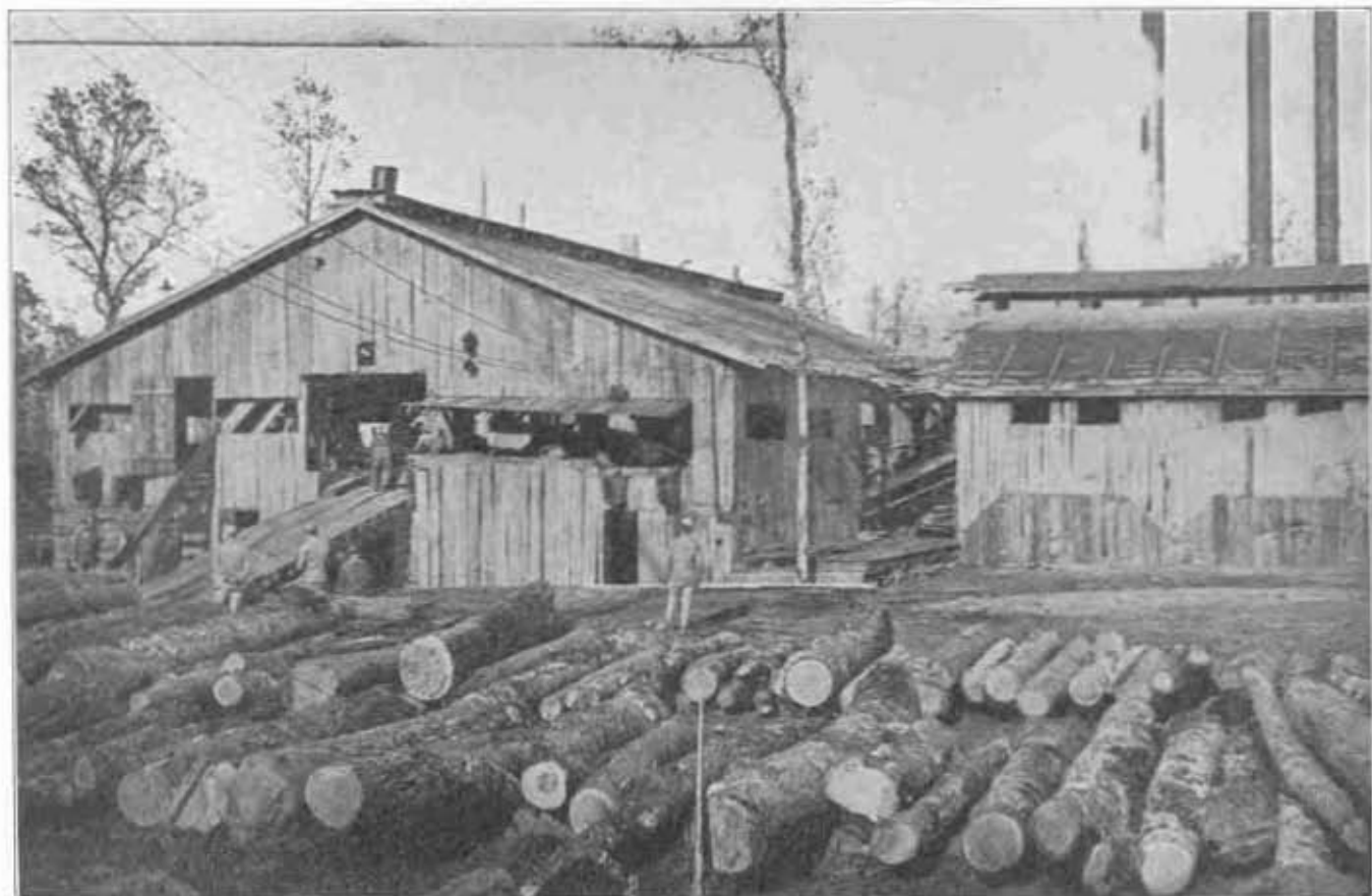
THIS WAS ERECTED BY THE 20th ENGINEERS NEAR ST. DIZIER AND SURPRISED THE FRENCH WITH ITS LARGE DAILY PRODUCTION, AS IN FACT DID ALL THE OTHER MILLS
