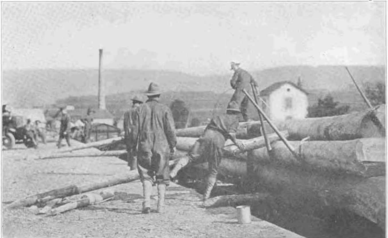
23th ENGINEERS LOADING LONG PILING FOR SHIPMENT FROM EASTERN FRANCE TO BASE PORTS ON ATLANTIC COAST TO BE USED IN DOCK CONSTRUCTION
