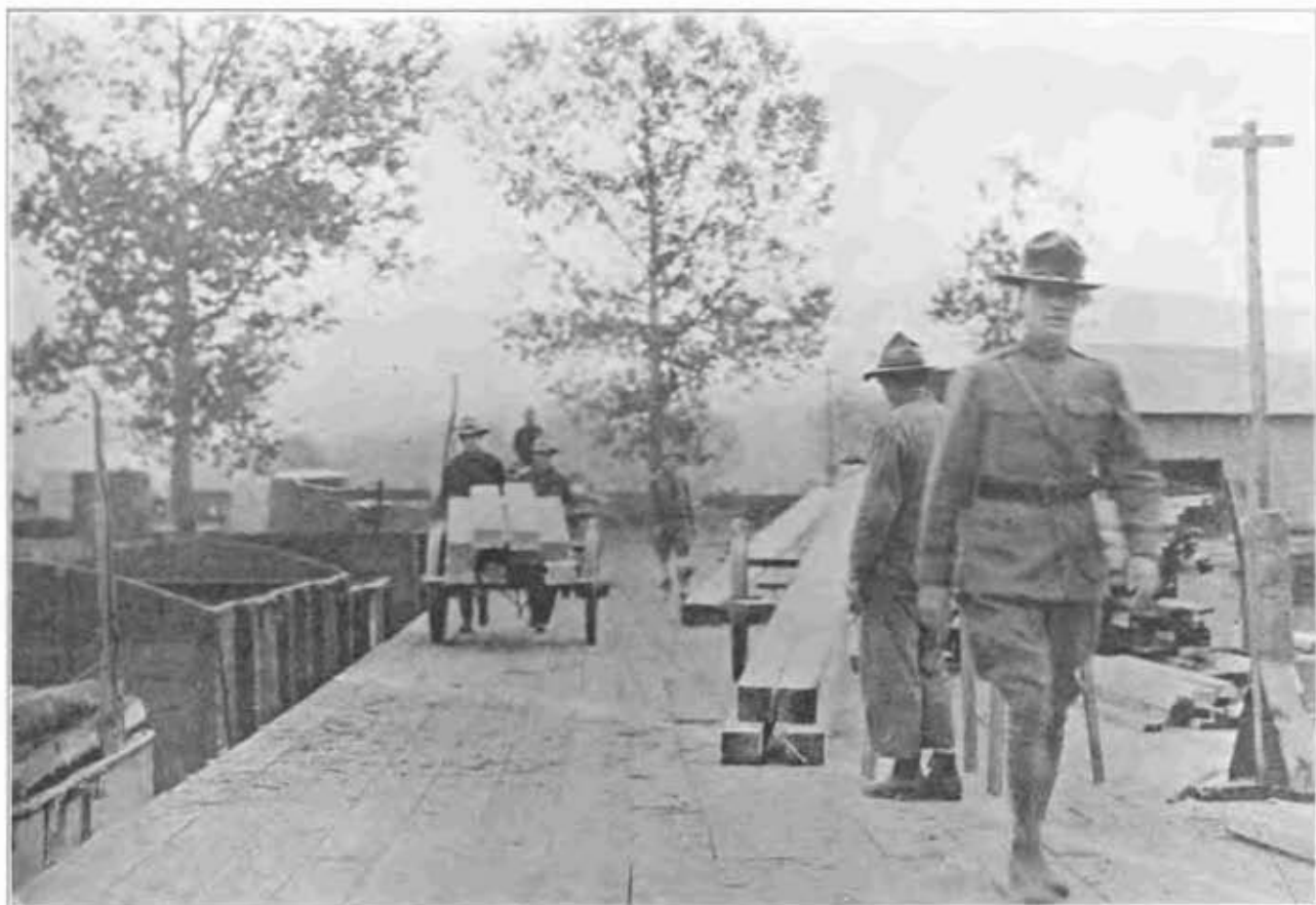
LOADING SOME OF THE MANY THOUSANDS OF TIES MADE BY THE 20th REGIMENT MILLS FOR THE A. E. F. OPERATIONS IN FRANCE
