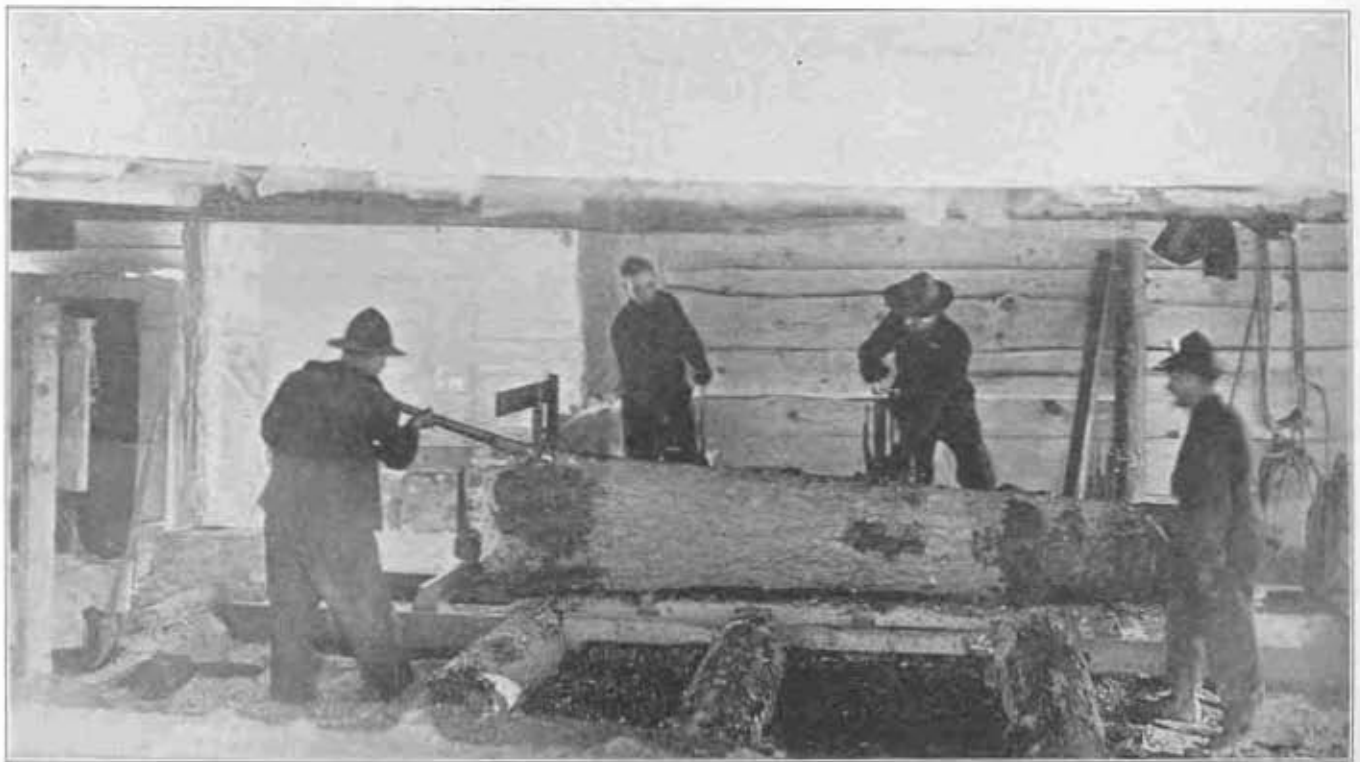
INTERIOR OF 20th ENGINEERS SAWMILL IN FRANCE
