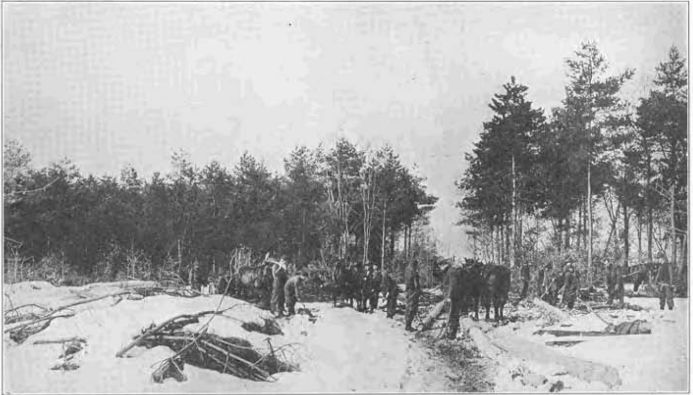
20th ENGINEERS SKIDDING AND PEELING POLES IN A FRENCH PINE FOREST IN SOUTHWESTERN FRANCE
