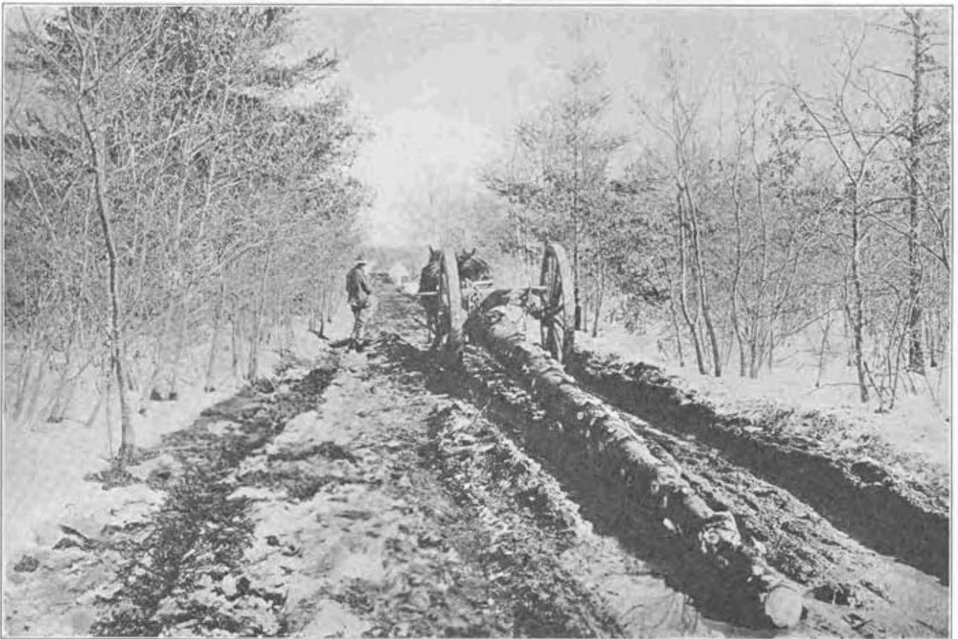
20th ENGINEERS IN FRANCE HAULING A SPRUCE TREE FULL LENGTH BY MEANS OF BIG WHEELS FROM WOODS TO MILL. OAK COPPICE AT THE SIDES OF THE ROAD.
