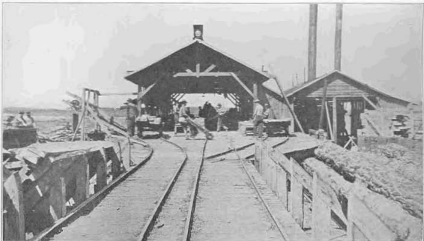
THE AUREILHAN 20-M AMERICAN SAWMILL NEAR PONTENX, LANDES, FRANCE, SHOWING THE SYSTEM OF TRACKS UPON WHICH THE TIMBER AND LUMBER ARE REMOVED FROM THE MILL TO BE LOADED DIRECT TO THE BROAD GAUGE RAILWAY CARS
