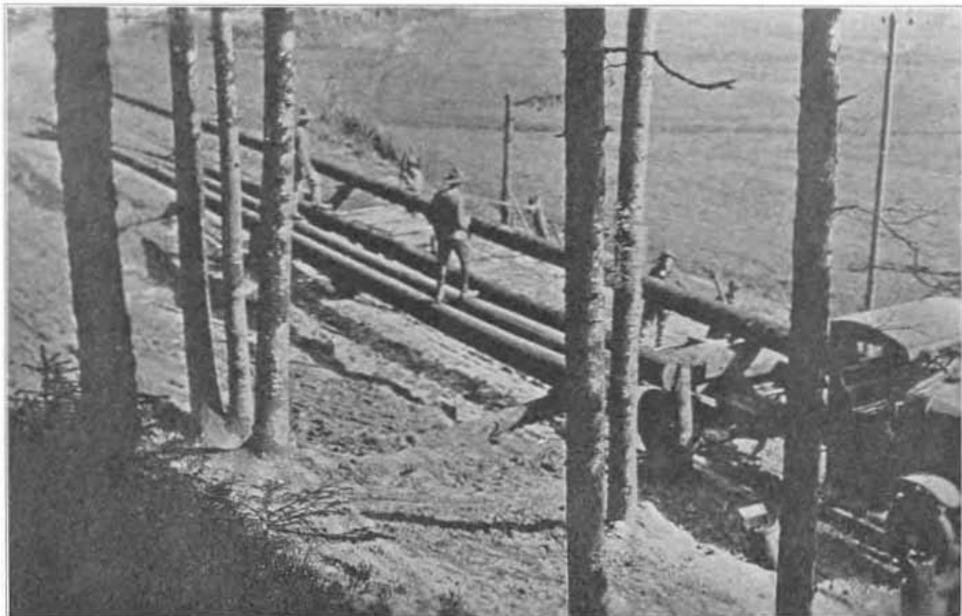
MEMBERS OF THE 20th ENGINEERS LOADING PILING ON TRUCKS AT LANDING No. 2 IN FRANCE. THESE PILING ARE APPROXIMATELY SEVENTY FEET LONG
