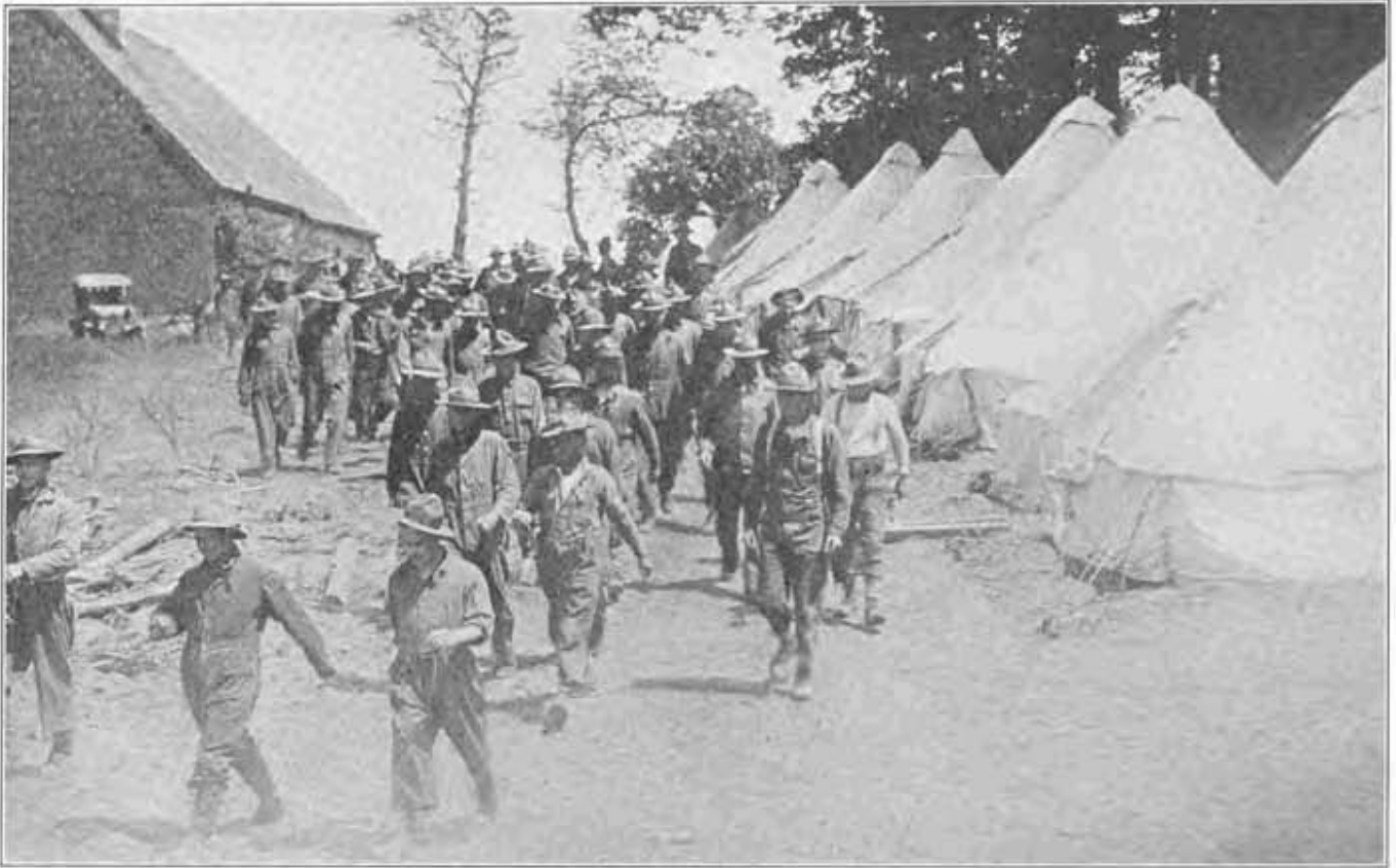
CAMP OF DETACHMENT OF 20th ENGINEERS IN FRANCE. CREW STARTING TO WORK
