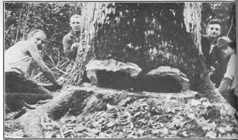
FELLING LARGE OAK, CIEZ COULOUTRE
