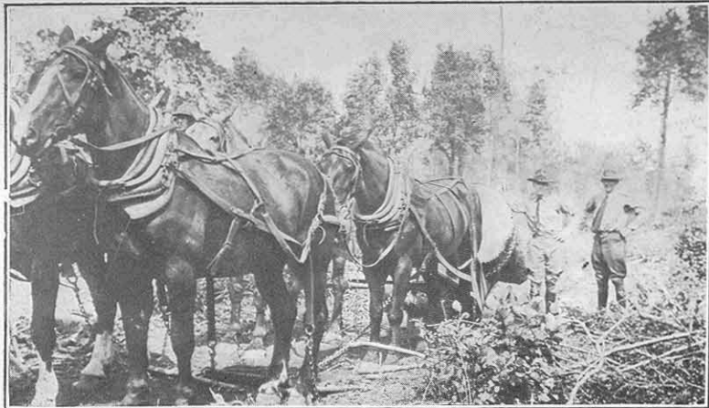
SKIDDING WITH SPOOL SKIDDERS, JULIAN OPERATION
