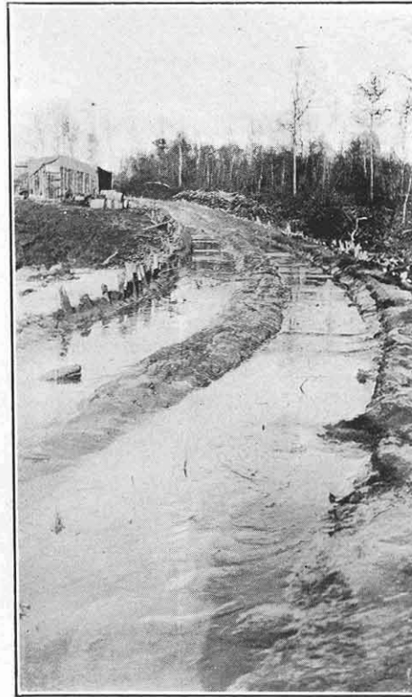
TYPICAL MUDDY ROAD CIEZ COULOUTRE
