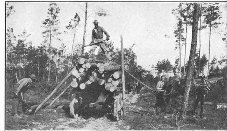
LOADING LOG WAGON WITH CROSS-HAUL
