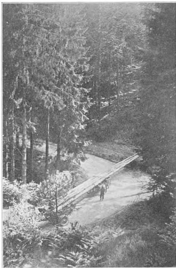
A LOAD OF PILING APPROXIMATELY 70 FEET LONG ON MOTOR TRUCK AND TRAILER GOING AROUND SHARP TURN IN THE ROAD IN A FRENCH SPRUCE FOREST. OPERATIONS OF 20th ENGINEERS
