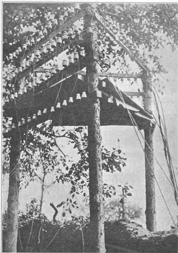
THE LUMBERJACKS AND FORESTERS HELPED TO BUILD TELEPHONE SYSTEM PLATFORMS IN FRANCE WHICH WERE LIKE FIRE LOOKOUT STATIONS IN OUR OWN FORESTS.
